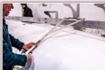
Marking stations on hull
